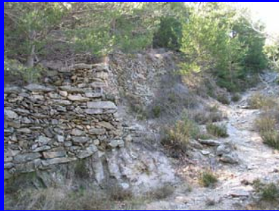
Linear erosion along a path in sandy soils.
